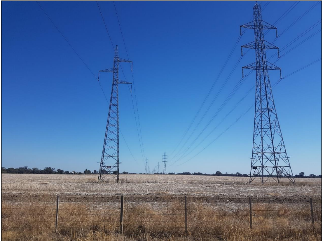
Eastward view from Boundary Road along the alignment of high voltage transmission lines
