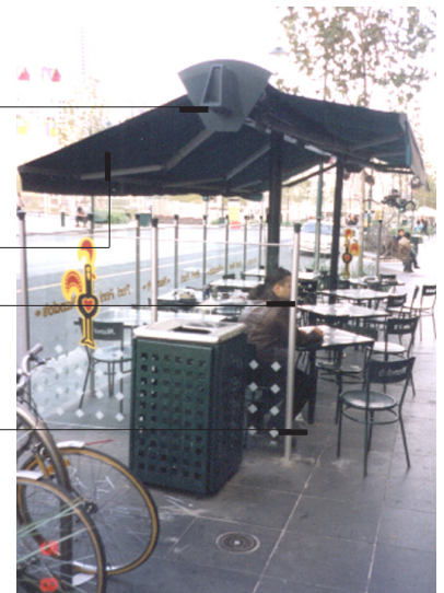
Permanent Shade Structure
