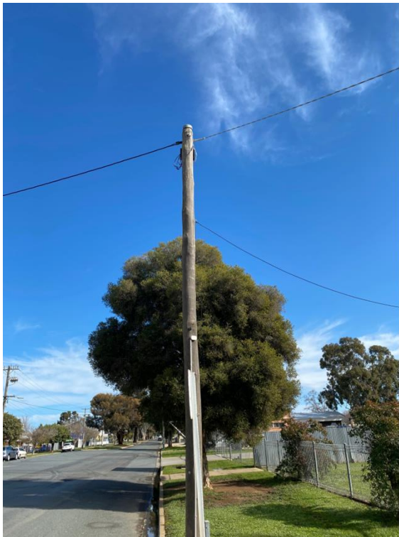
Existing power pole in Casey Street nature strip which provides overhead connection to a dwelling that is to be demolished.
