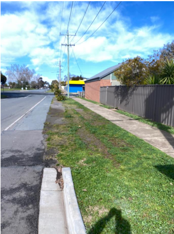
View of Albert Street which has no kerb and channel
