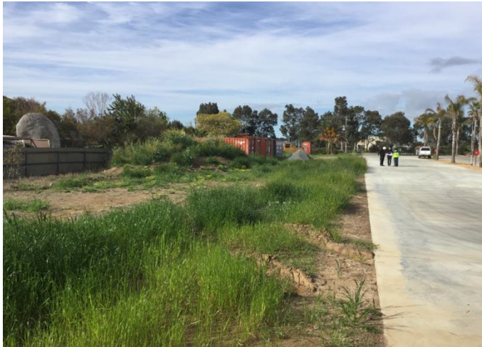
View of the development site looking south towards Kialla Lakes Drive
