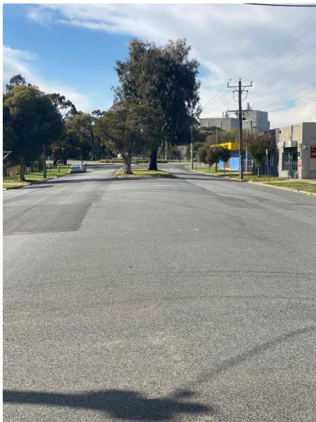
View of Casey Street looking towards TMI
