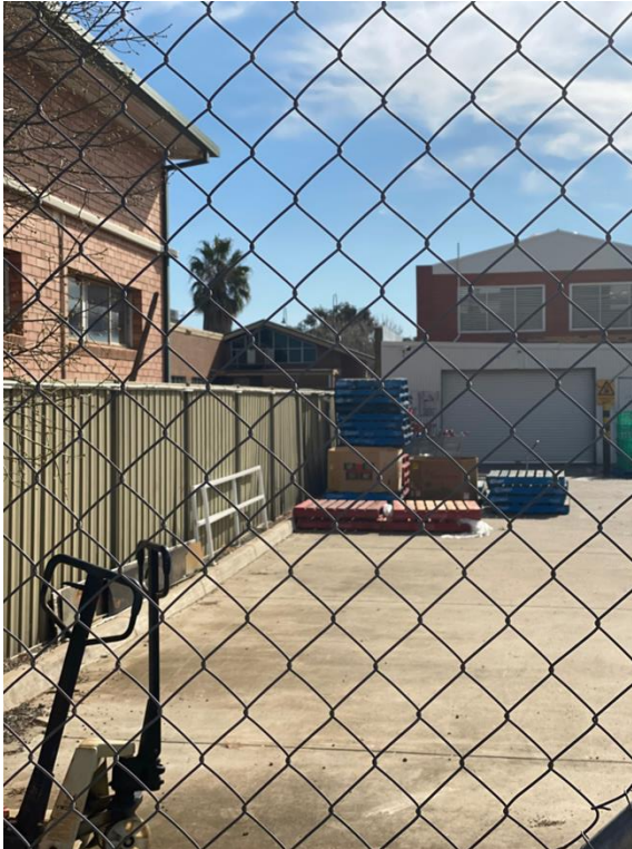
View of boundary fence on the lands western boundary to the Telstra Exchange
