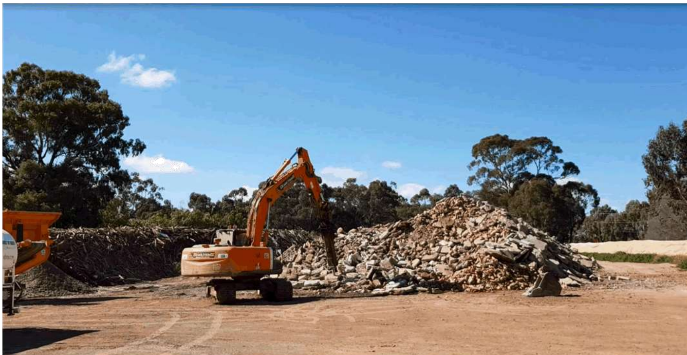
Photo taken during rock breaker trial
