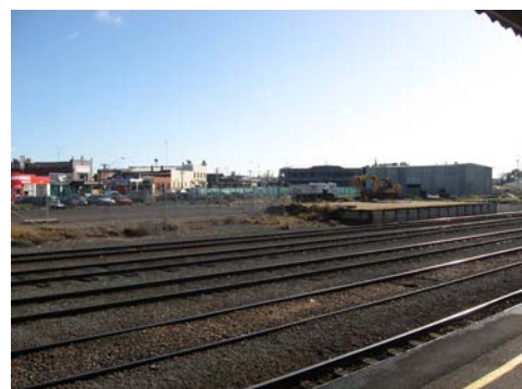
Looking towards the CBD from the platform of the Shepparton railway station. A new link from the station platform through to Hoskin Street will provide a direct pedestrian route to the CBD and High Street..
