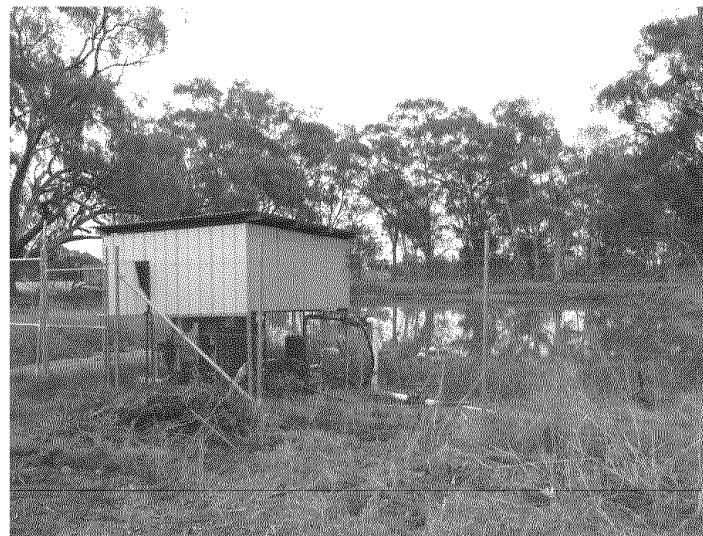
Figure 24: Dam and pump shed
