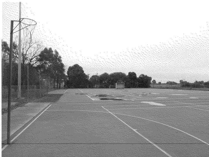
Figure 9: Netball / Tennis Courts
