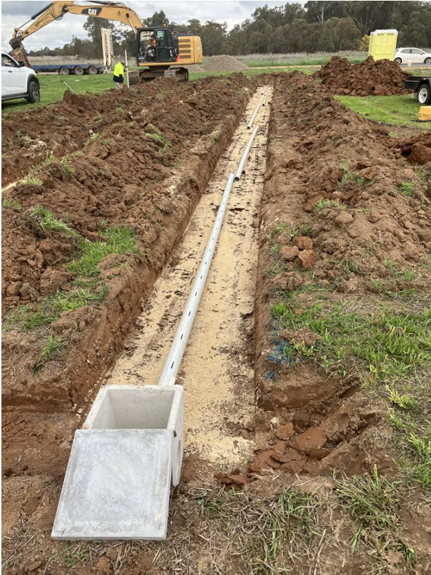
Image 12: Evapotranspiration trench with gypsum sprinkled along the bottom of the trench. Trench is 400mm deep and 1m wide
