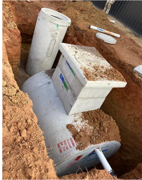
Image 8 – Septic tank with riser lids finished at ground level. All waste septic tank with risers extended to ground level to ensure access for pump out and other maintenance. Pump well installed at the outlet of the septic tank to pump to effluent disposal trenches.
