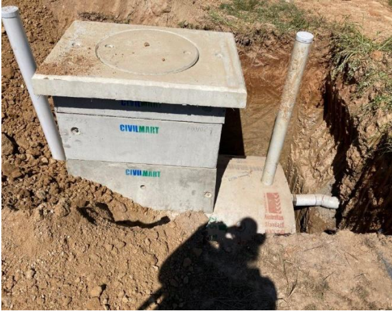
Image 8 – Septic tank with riser lids finished at ground level. All waste septic tank with risers extended to ground level to ensure access for pump out and other maintenance. Pump well installed at the outlet of the septic tank to pump to effluent disposal trenches.
