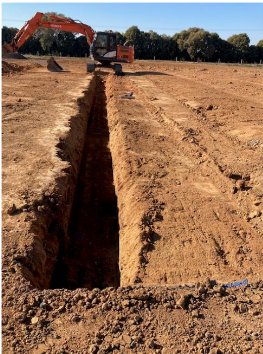
Image 17: Excavation for a Wick Trench
