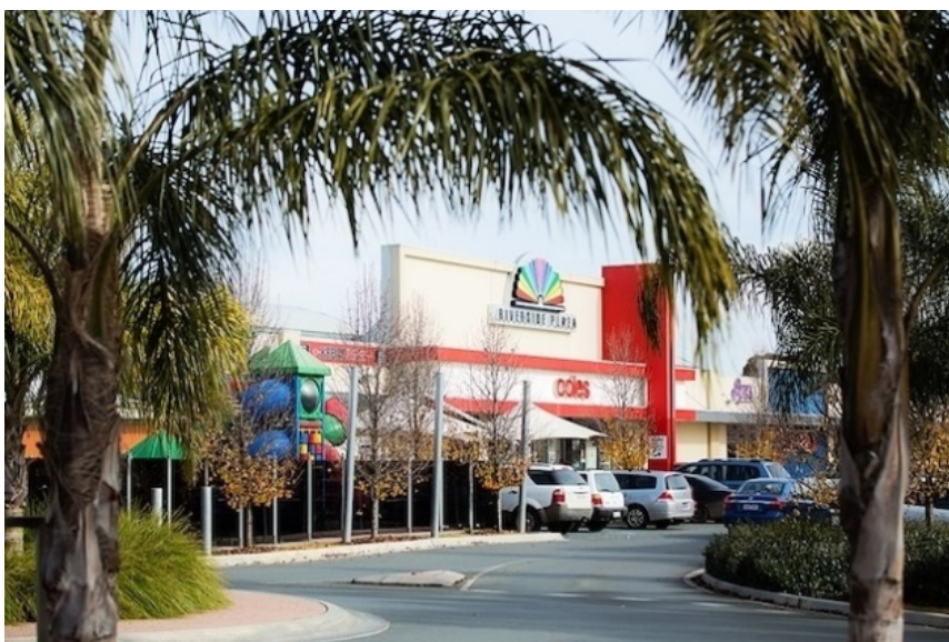
Picture: Shade structures over car park at Riverside Plaza, Kialla
